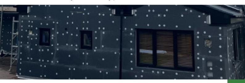
The mechanical fixings used can be seen in the photo below. When using 90mm-100mm thick EPS, the fixings required are 140-170mm long.
